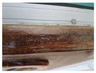
**Rob** also told the story of using epoxy resin as a varnish on timber. Initially it looked superb but due to its poor UV resistance its appearance didn't stand the test of time.
