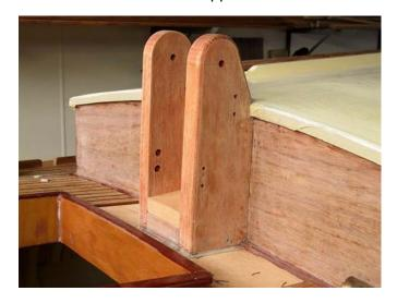
The deck is Burmese teak glued straight to the ply decking. Clive noted the need to wash the teak thoroughly with acetone to remove the natural oils near the surface and apply the glue quickly before the natural oil comes back to the surface. This process was
