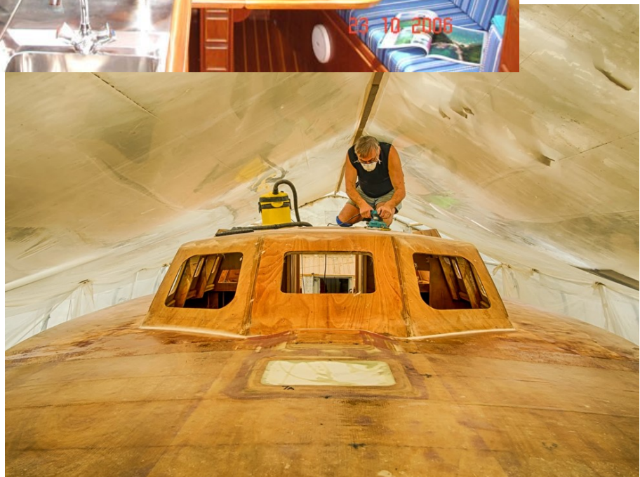
AN MC36 BEING BUILT IN NEW ZEALAND
