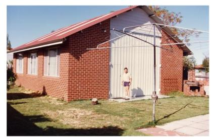
By 1991, work on Argosy was put on hold whilst Chris built a purpose designed shed at the back of his house in Wembley. This is more the shed that has the house in its front yard! It has an 80 square metre floor, double brick construction and 5.5 metre high steel portal frames. Apart from specialist trades such as the grano, steel, brick and electrical work, Chris completed the details himself including manufacture of the large doors each end and the associated heavy duty hinges.
