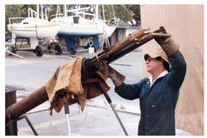
A small frame was used to provide support to the short ribs in the top end of the bore casing — primarily in the steam rather than the boiling water.
