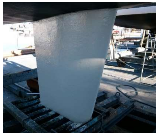
Applied Hempel two pack epoxy primer & undercoat directly to the shiny metal. ( Hempel Light Primer & Curing Agent 95360 Ratio 2:1) No time to fill and sand so some divots remained. No time to give keel to hull joint much attention so expected this to be a rust area next time boat was slipped.
