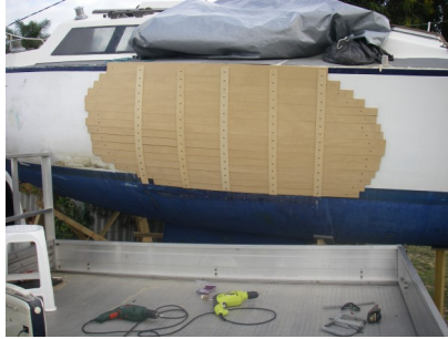
Cutout marked on inside
