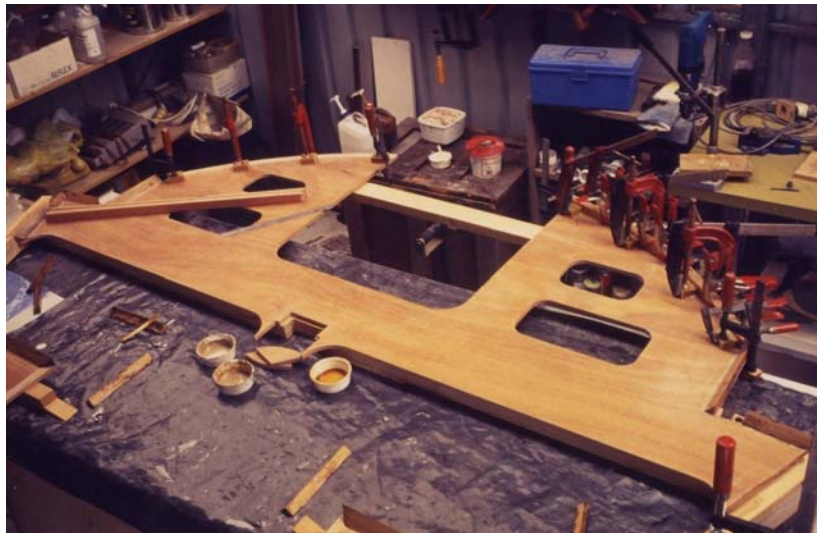
Each bulkhead was fully made up in the workshop before any assembly proceeded
