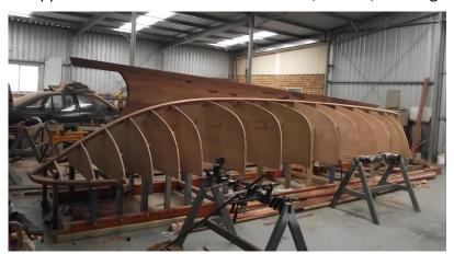
Currently the stem and keel have been fitted and all the frames set up. The skeg is temporarily fitted to facilitate planking, but will be removed to allow sheathing, then will be
