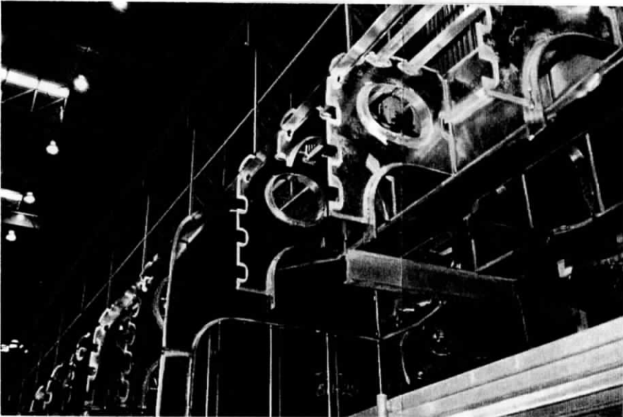
Close-up of some of the frames and part-frames. Grinding and cleaning along all edges where welding is due evident.
