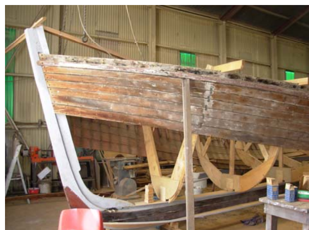
Internal frames to maintain Kiewa's shape, some planks reattached—halfway through the work at Fremantle Boat Manufacturers
