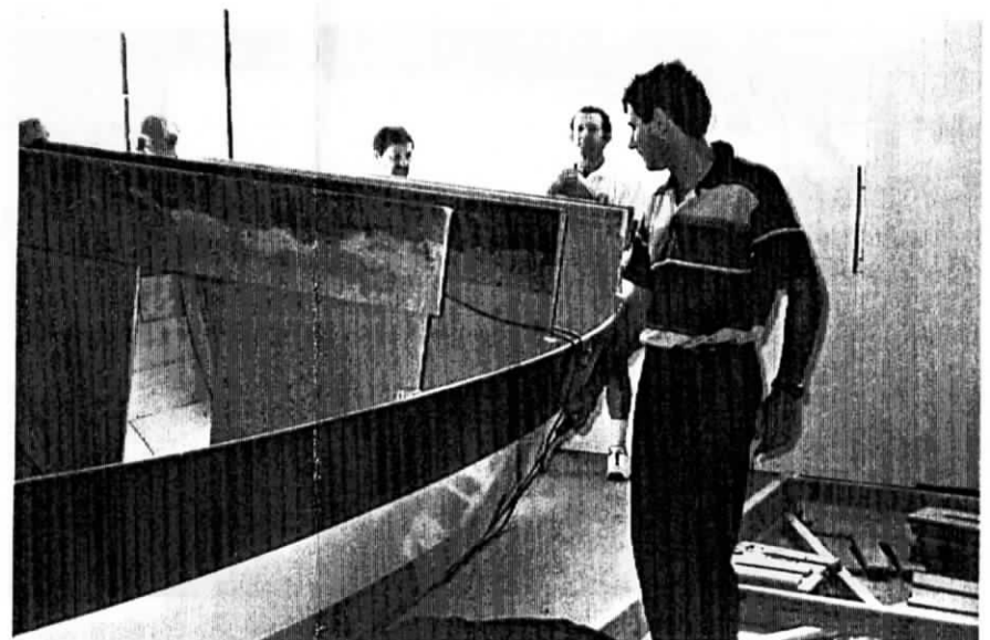
John McKillop takes the strain on one lifting strap to lift her back over the building jig.
