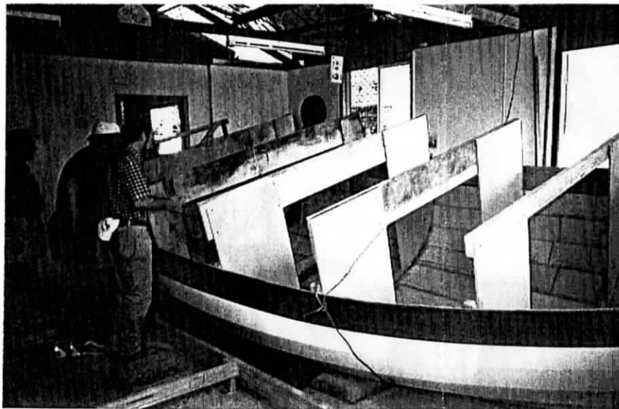
Ready for the lift back over the jig. All the temporary frames can be clearly seen.
