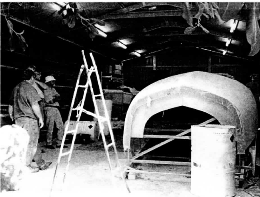
ABBA members in foreground explaining to Mark that they forgot to bring their old clothes to assist with fairing. Illustrates scale of shed and vessel.
