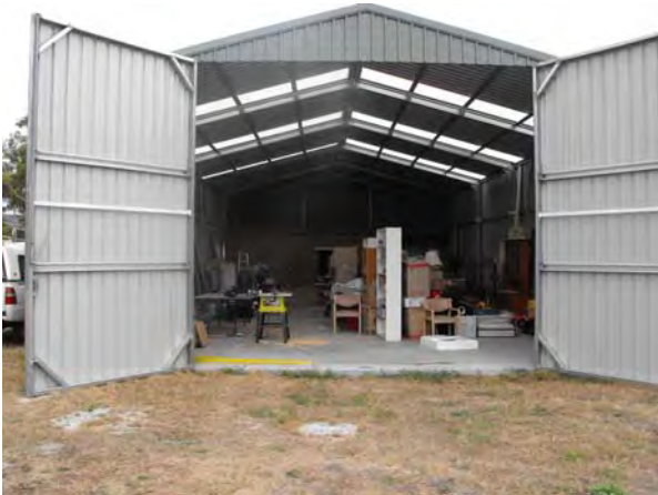
A large shed for a large project
